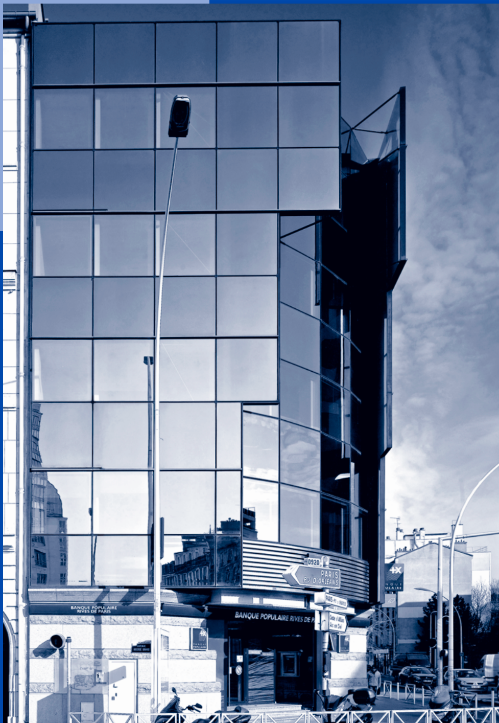
Montrouge (92) 55 avenue Aristide Briand
